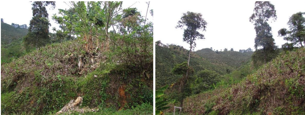
Figure 10 and Figure 11 Landscape of Tunnel Tesalia Exit
