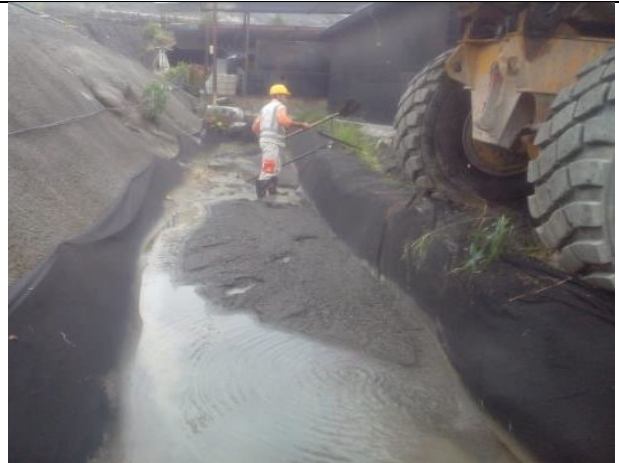
Maintenance of run-off channels in La Sorda exit portal – UF7
