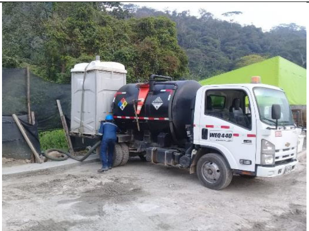
Maintenance of mobile sanitary units in UF7
