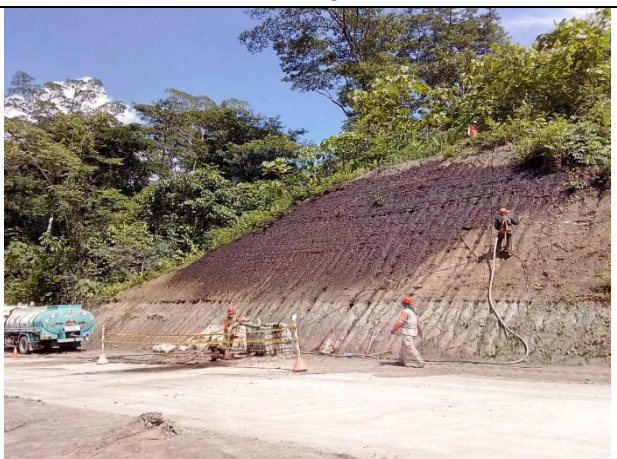
Slope protection on roadworks by hydroseeding – UF5
