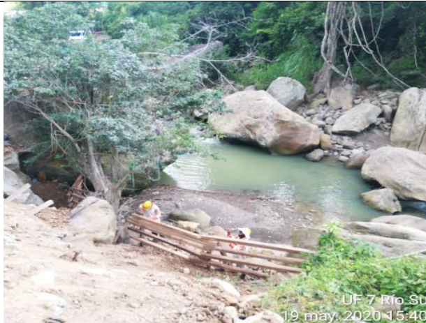
Riverbed protection in Río Sucio - UF7
