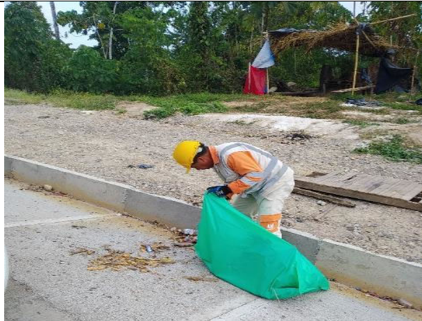
Waste management- drainage clearing in UF3-4
