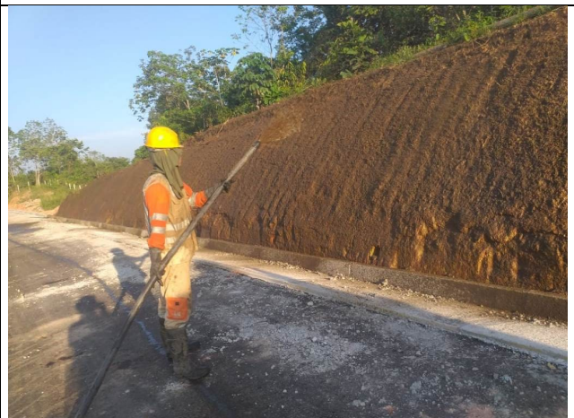
Slope protection by hydroseeding
