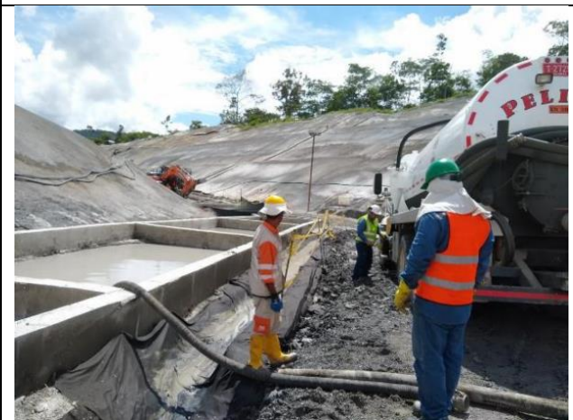
Water treatment of tunnel excavations
