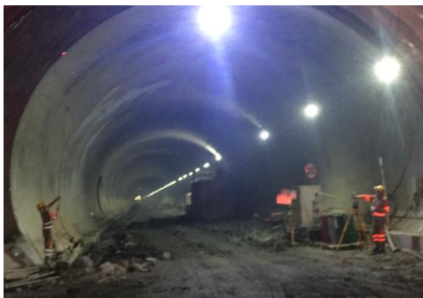
Finished excavation activities in Mulato Tunnel
