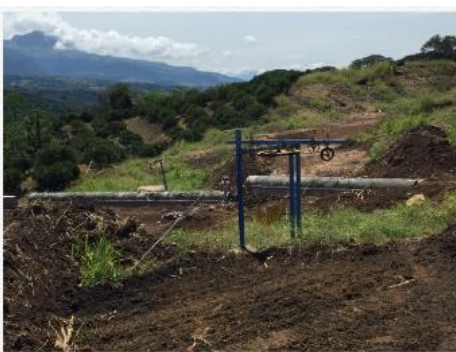
Peña Bonita Property – Works activities for protecting the productive project
