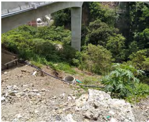
Flow monitoring in Tunnel Mulatos
