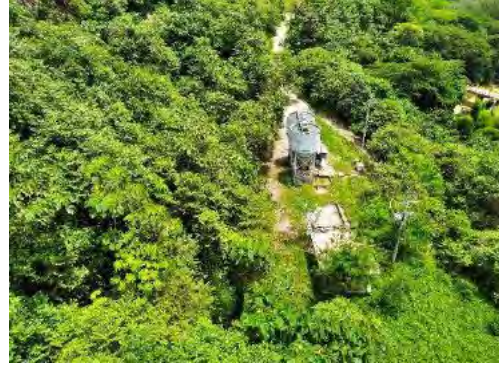
WWTP Tunnel Mulatos
