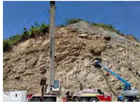
Slopes stabilizations in UF 2
