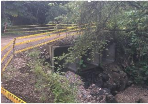
Punitive Action Box Culvert Area, no damages or risks identified
