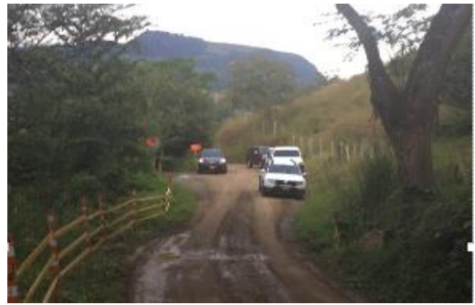
Punitive Action Industrial Roadway Area, no damages or risks identified
