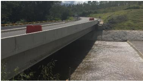
Finished water occupations in UF 1
