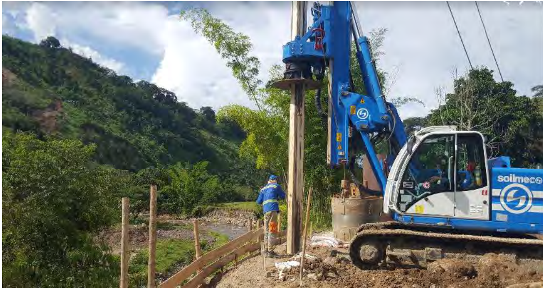
Image 6 Adequate water course protection
