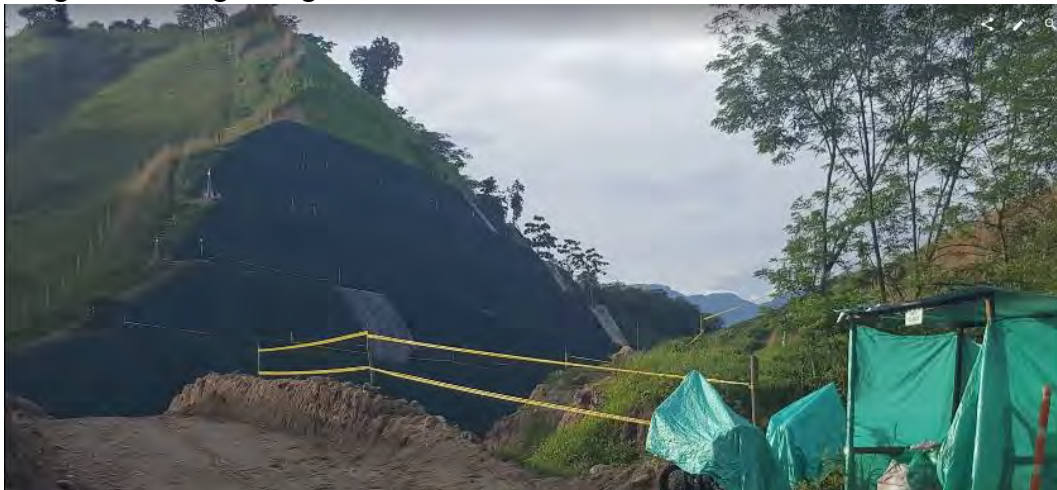
Image 4 Adequate planting of vegetation cover in slopes
