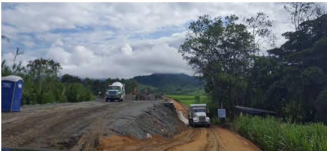
Image 8 Earthworks in UF1
