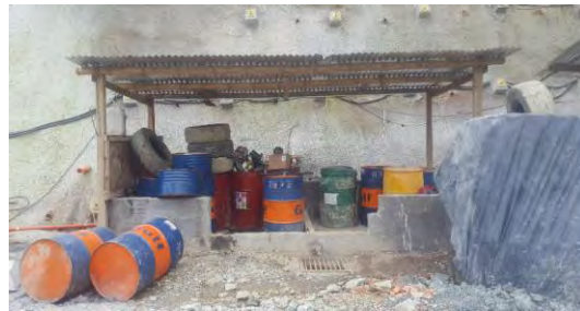
Figure 2 Overcapacity storage of hazardous materials
