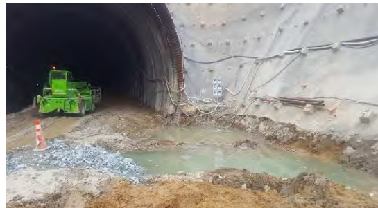
Figure 8 Tesalia Tunnel Entrance
