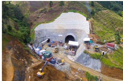
Figure 4 Exit portal of the La Tesalia Tunnel
