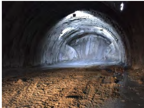
Figure 20. Advance in construction activities Tesalia exit portal.
