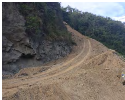
Figure 8 High slopes in Irra Tunnel, lifeline recommended.
