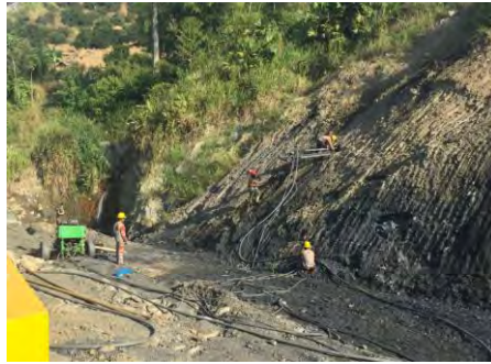
Figure 16 Stabilization and hydraulic works.
