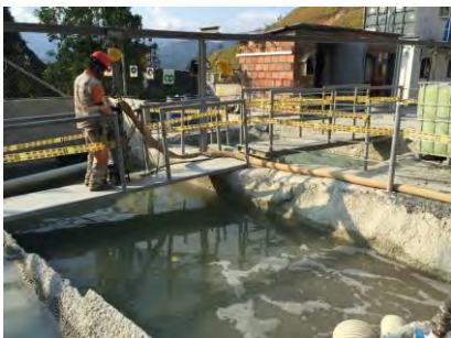
Figure 21. WWTP in Tesalia entrance portal.
