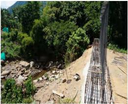
Picture 1 *La Ley* stream, K92+700, UF5. Lack of water protection barriers
