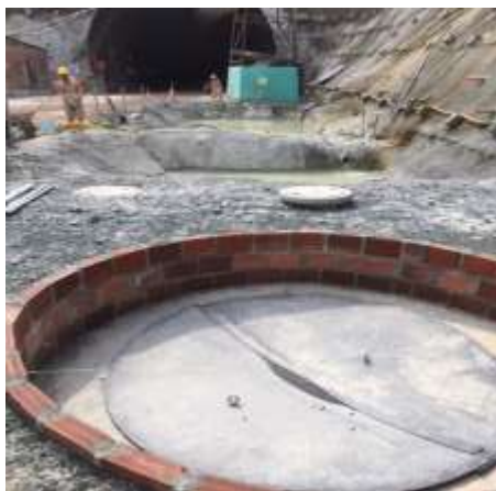
Figure 5 Sedimentation ponds at Tesalia tunnel – entrance portal
