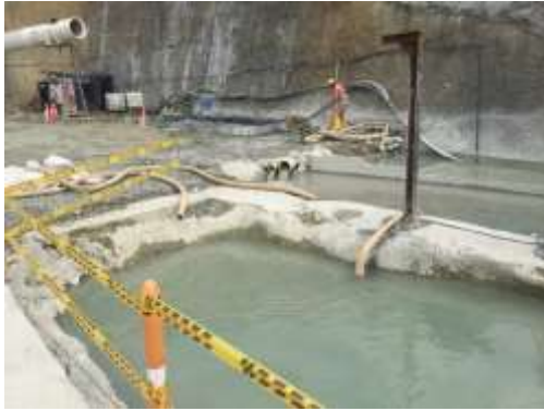
Figure 7 Sedimentation ponds at Tesalia tunnel – exit portal
