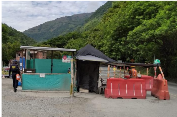
UF 5. Work fronts signaling and security
